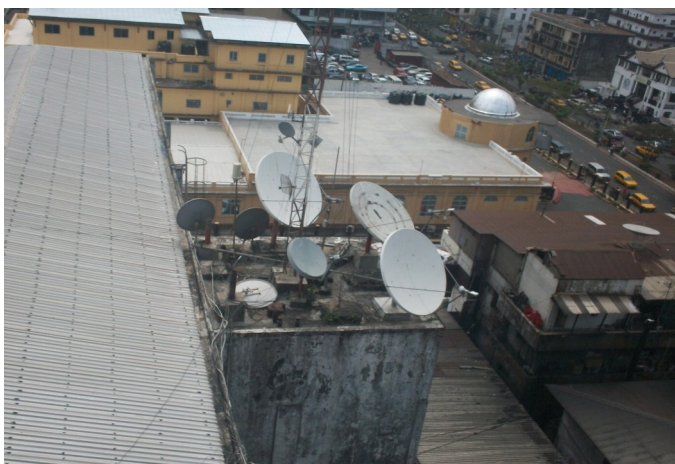
LTA Engineers collect telecommunications installation information in Central Monrovia in its Telecommunication Information Gathering Project
