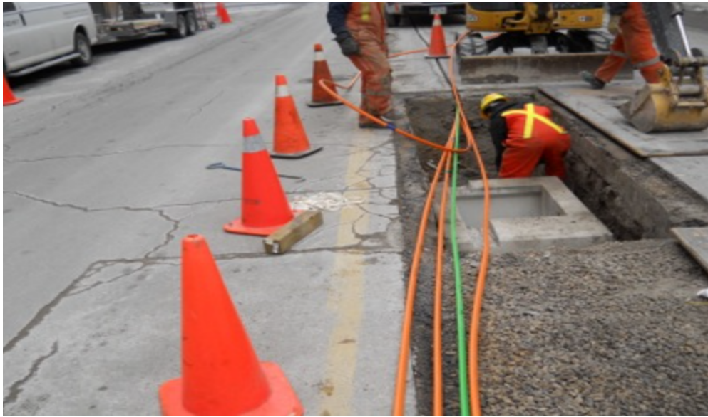
Figure 7. Mechanical Trenching Machine Laying Down Fiber
